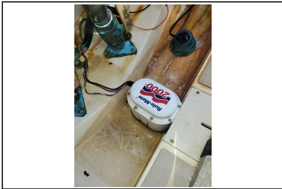
Bilge Pump AFT
