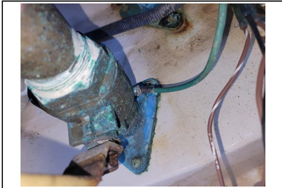
Bonding Wire at Thru-Hulls
