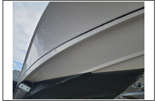
STBD Hull Side- pic 2
