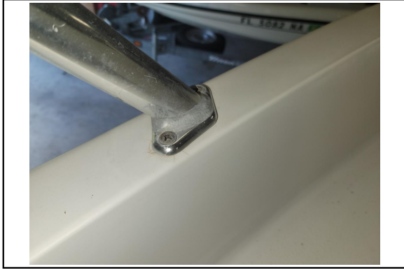
Bow Grab Rail-STBD Needs to be secured _085455
