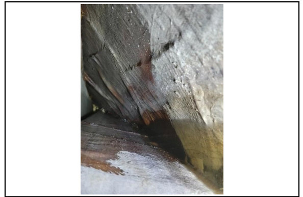
STBD Bow Stringer hull side
