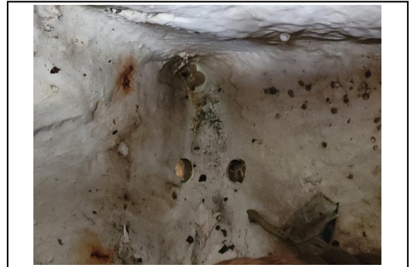
Limbol holes in the chain, anchor compartment
