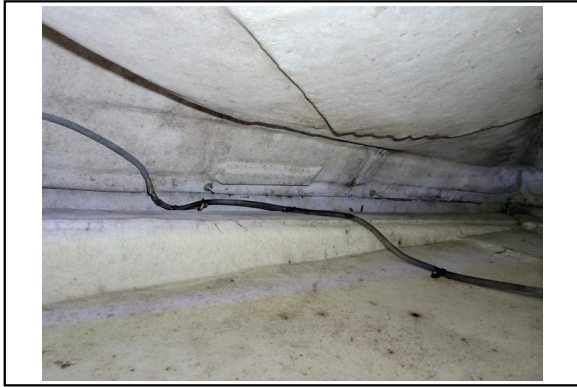
Hull to Deck Joint Bow STBD side
