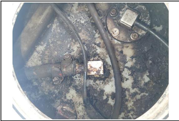
STBD Gas tank deck plate opening
