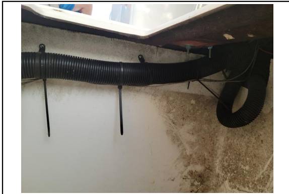
Secured and protected wiring
