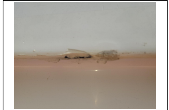
Gel-Coat Repair STBD side
